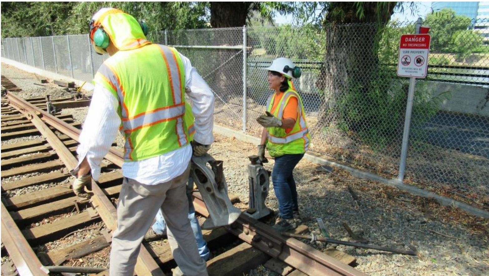
Steve and Pam deploy track-jacks for lifting the rail just enough to squeeze tie-plates beneath
