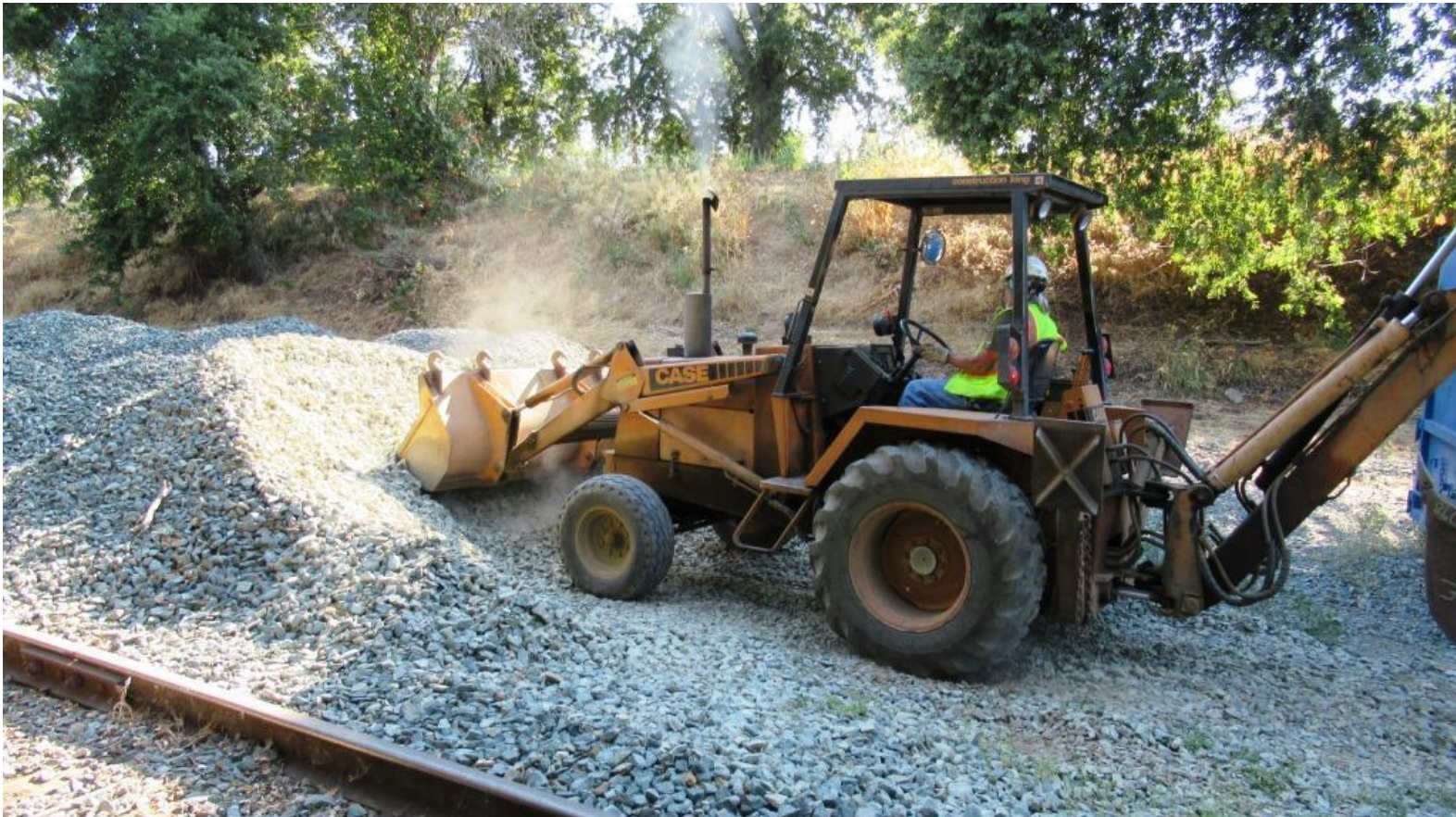
Ed, on the back-hoe, gets a big scoop of rock from our fresh ballast pile at Setzer...
