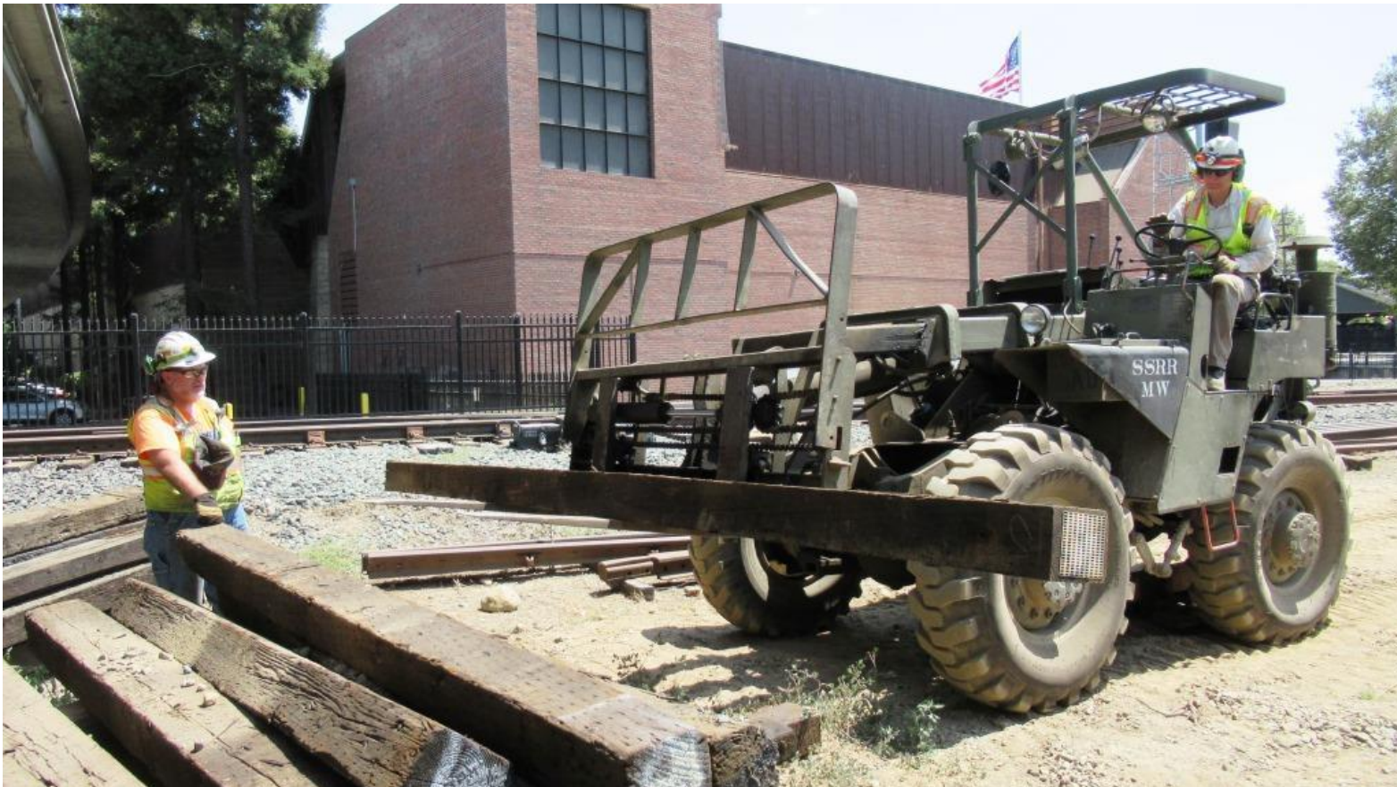
Mike F. works with Steve on Big Green to grab some extra-long switch ties from tie-pile
