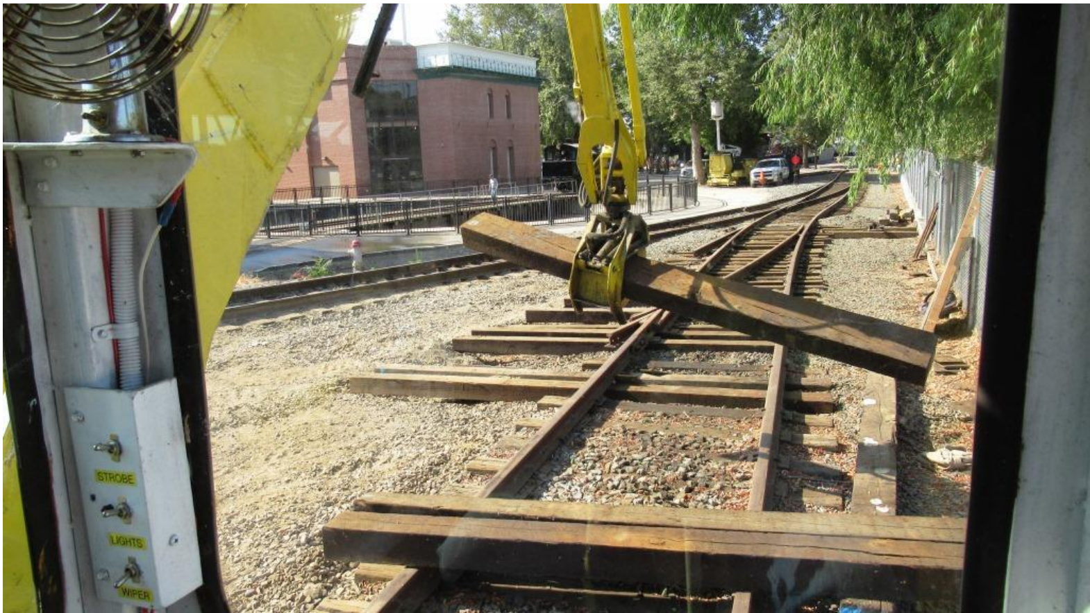
First up Saturday morning: moving the tie-crane and about six extra-long switch-ties sitting on the rails out of the way
