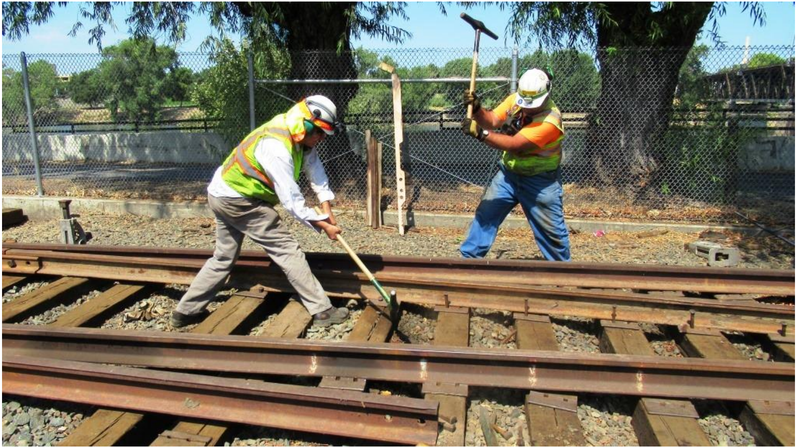
Steve and Mike F. demonstrate their world famous tandem windmill spike-driving technique
