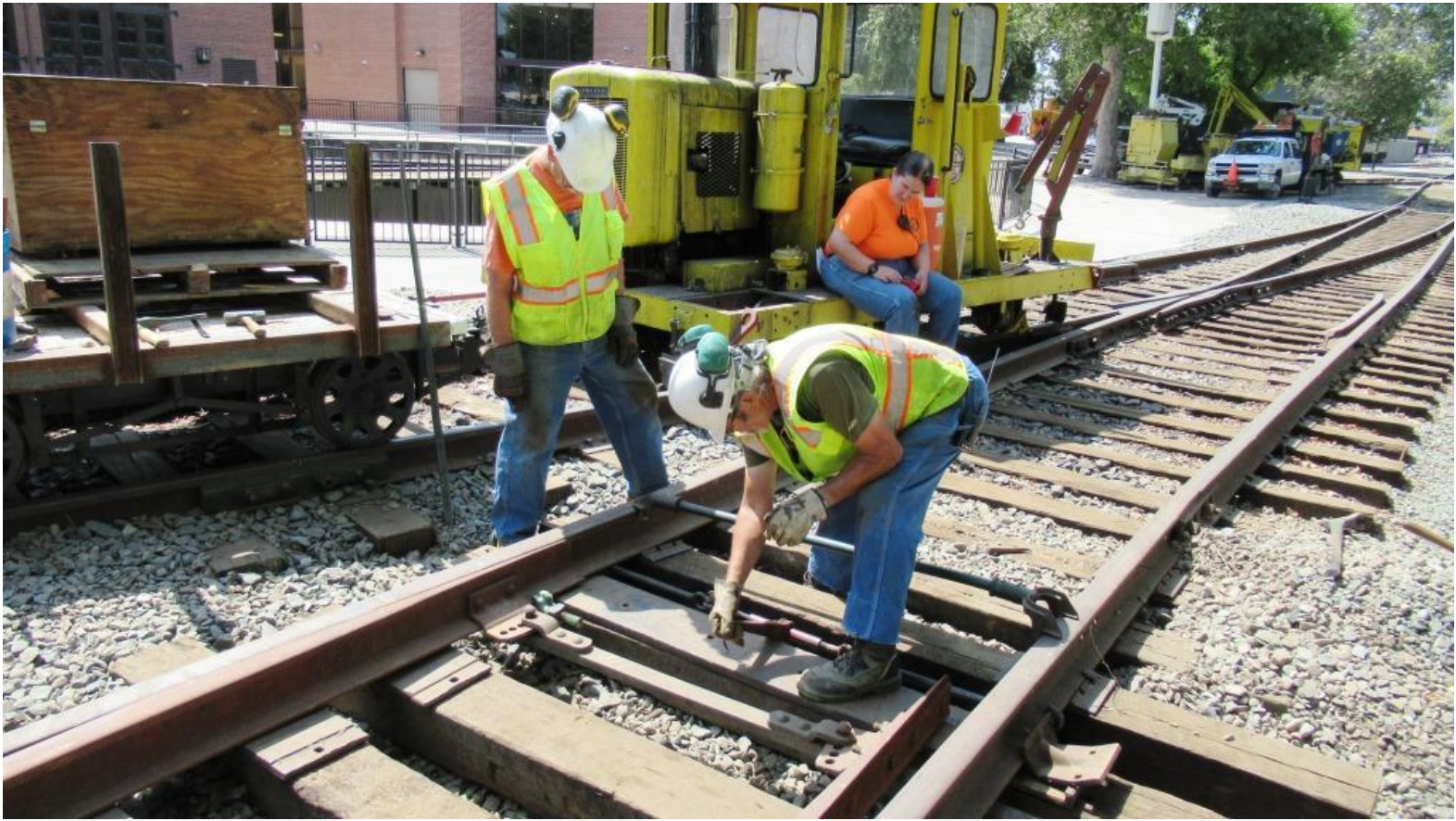
Ed and Clem use the grapple-gauger to fix the wide gauge issue near the switch-points
