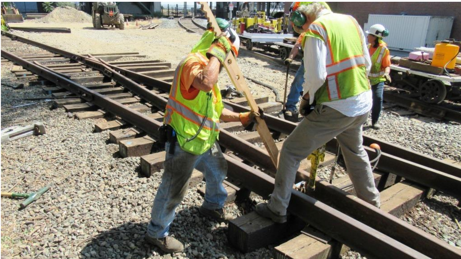
Joe now uses the Steve Tool to hold an unset spike for Steve to drive with the hydraulic spike-driver
