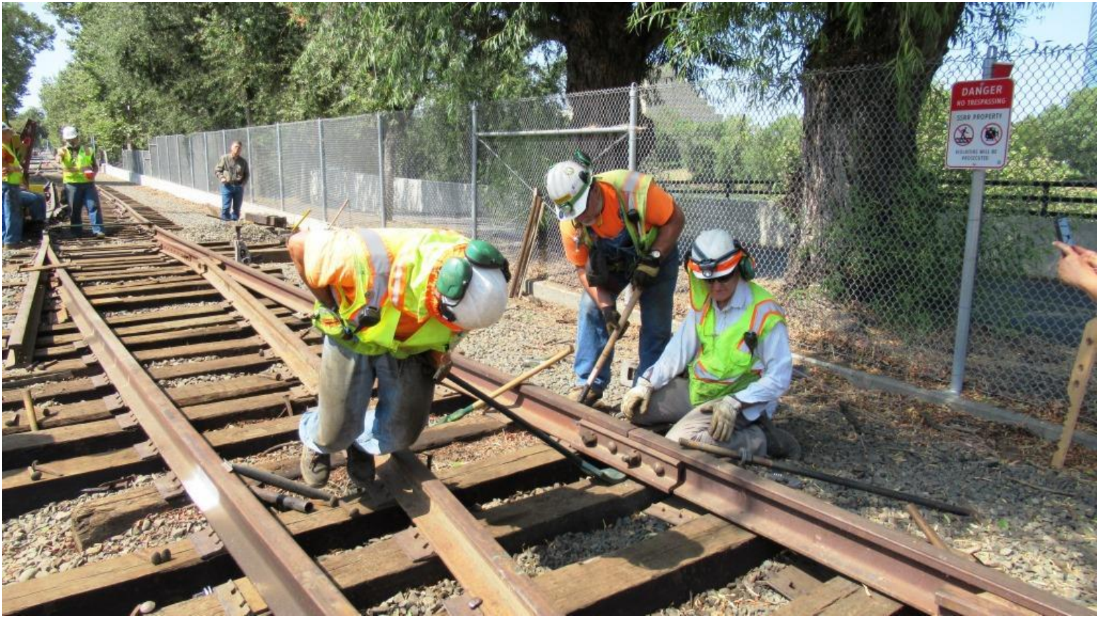
Joe puts his back and, well, whole body into nipping up the joint for plate insertion
