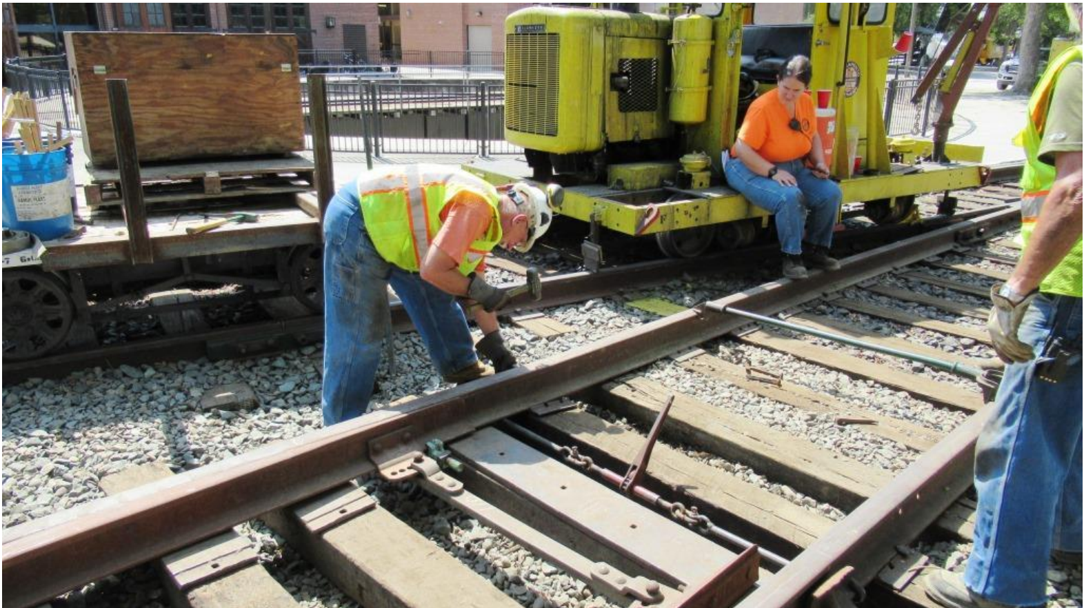
Then Clem sets spikes to hold the gauge
