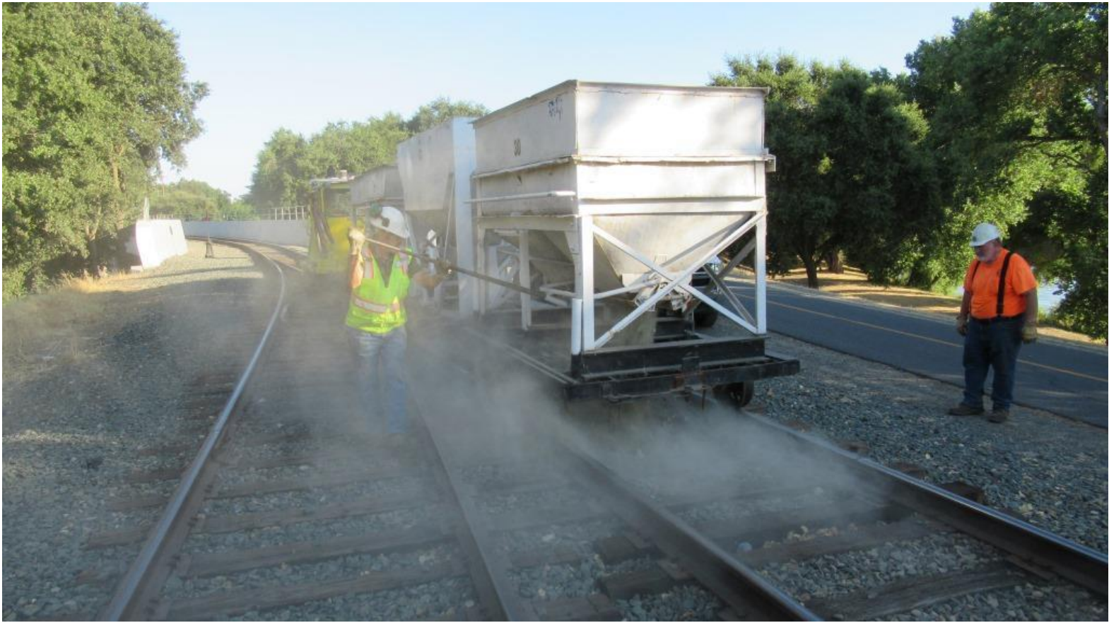
Ballasting began at Baths where Ed emerges from a fog to disgorge rock from the center-dump hopper
