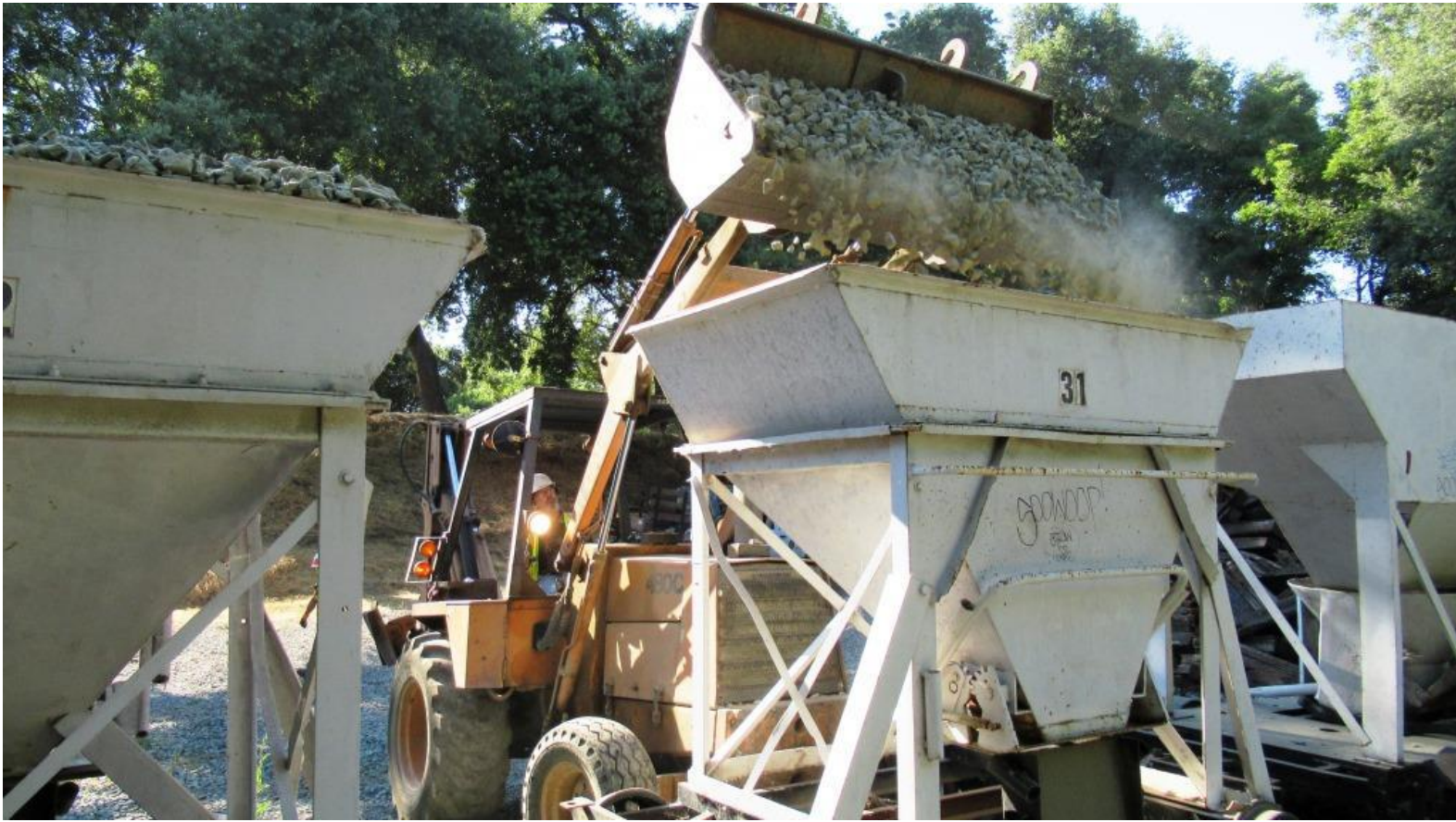
...And fills the ballast hopper cars with it
