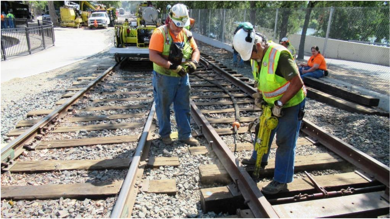
Ed drives home the spikes that were set to hold gauge at the switch-points
