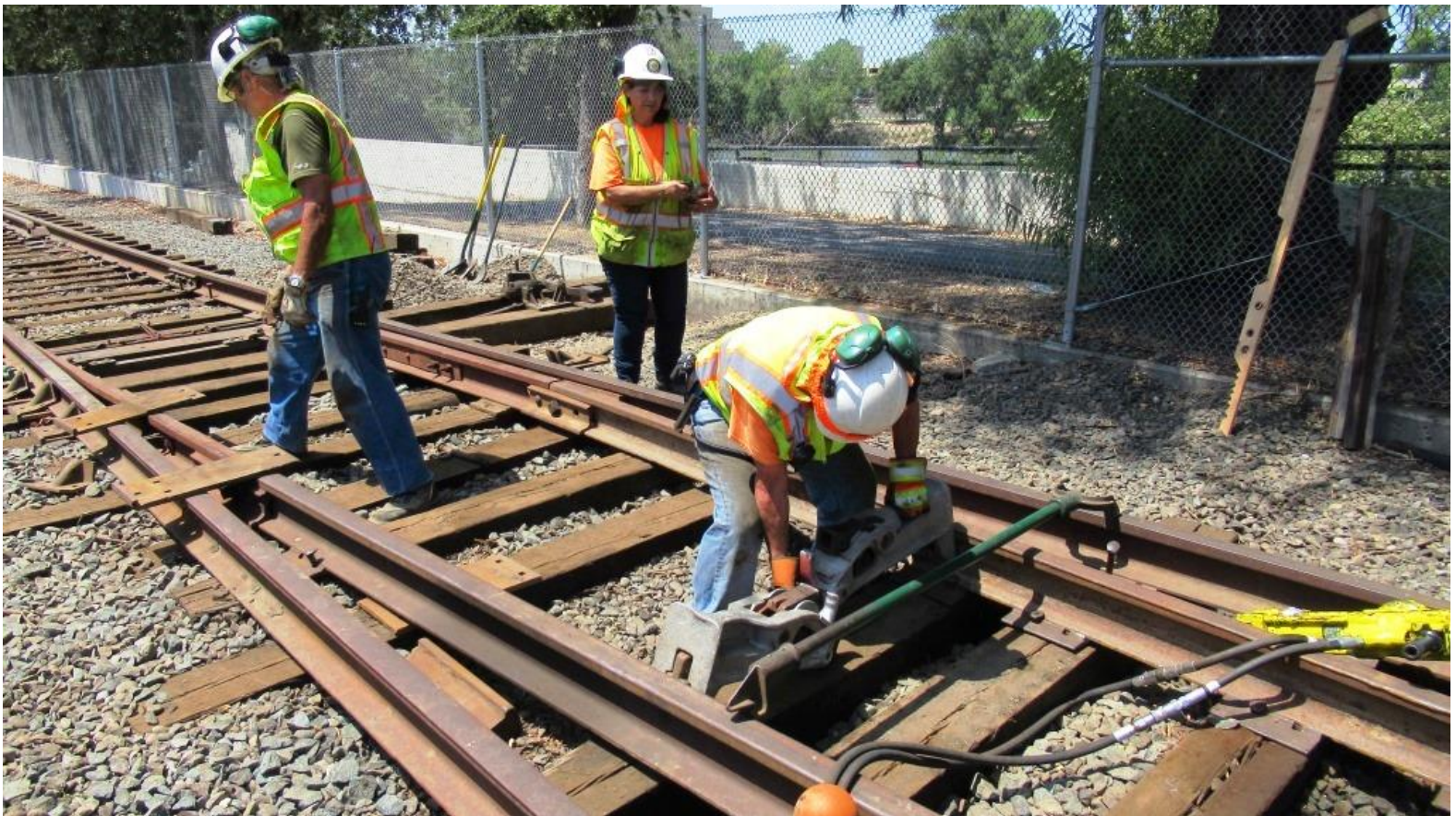
Joe places track-jacks horizontally to each other, to spread the rails where the gauge is narrow
