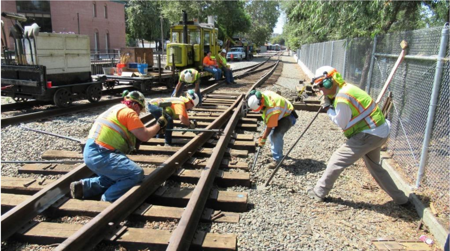
Your MOW Team at work: Mike, Pam, and Ed set spikes as Steve nips a tie that Joe hand-tamps some rock beneath
