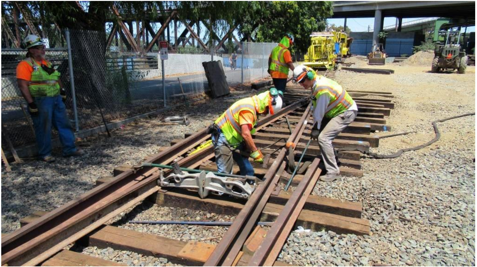
With the track now in gauge, Steve nips the rail as Joe sets a spike
