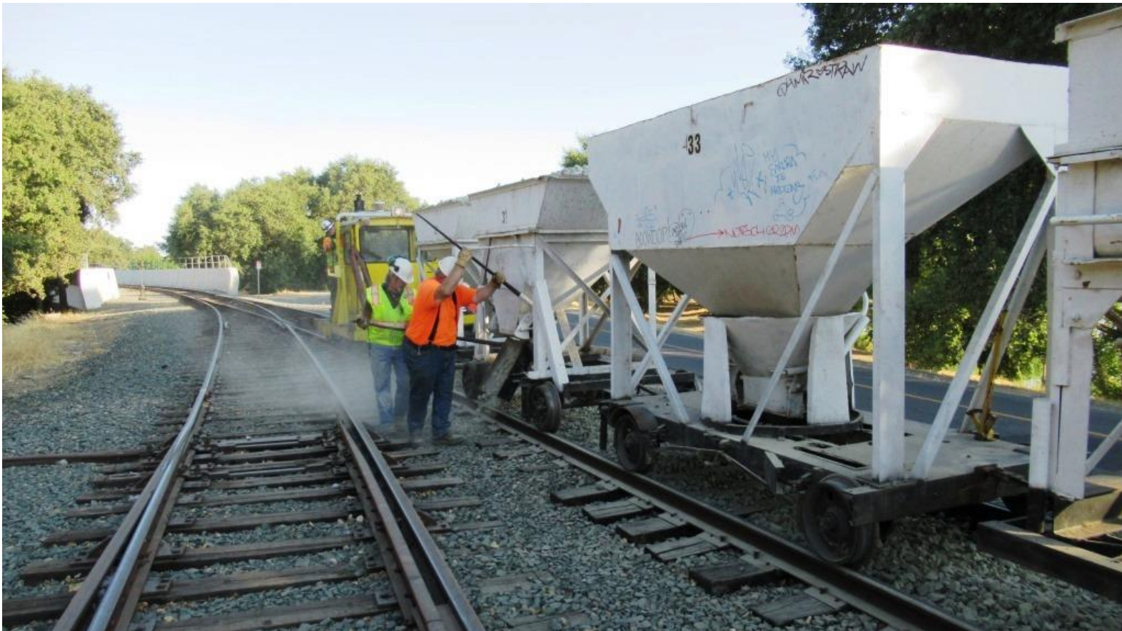
Frank and Ed now drop rock from one of the side-dump cars
