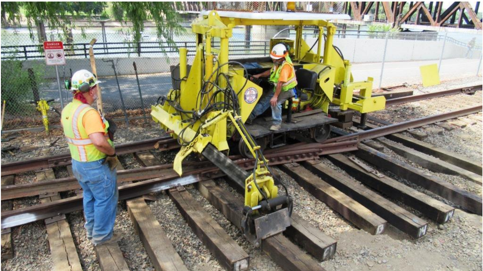
Joe brings in the Jackson 125 tie-exchanger to insert the long ties into the empty tie-cribs
