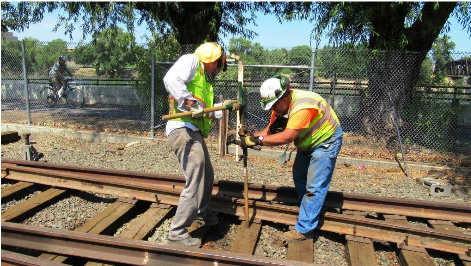
Steve and Mike F. use a spike and spike-maul to make field-repairs to another spike-maul
