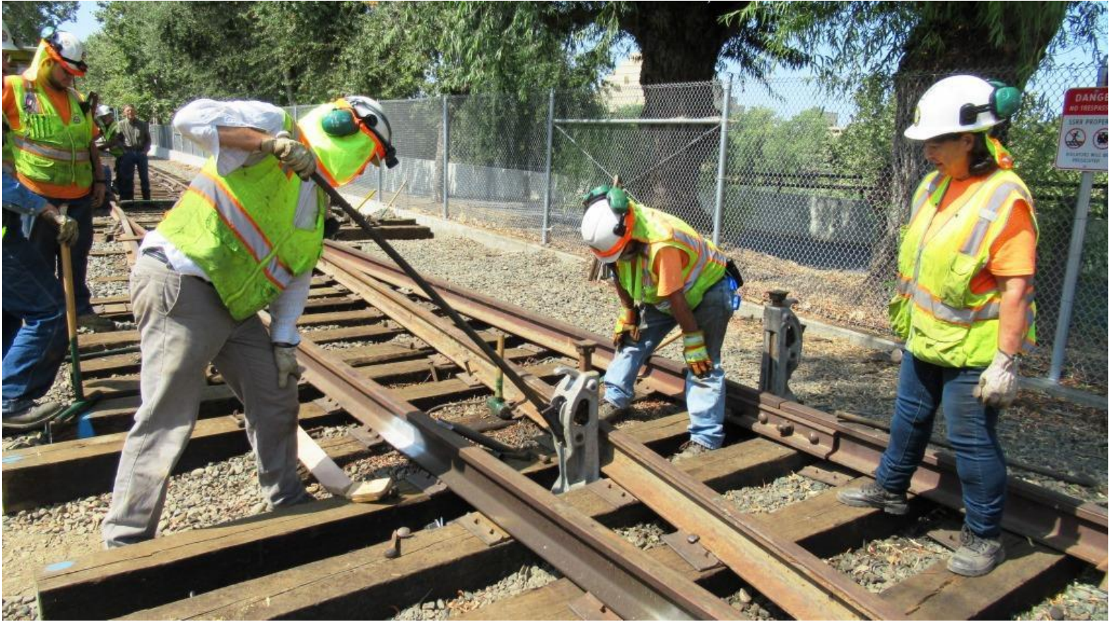
Steve cranks on the track-jack as Joe gets ready to set a plate
