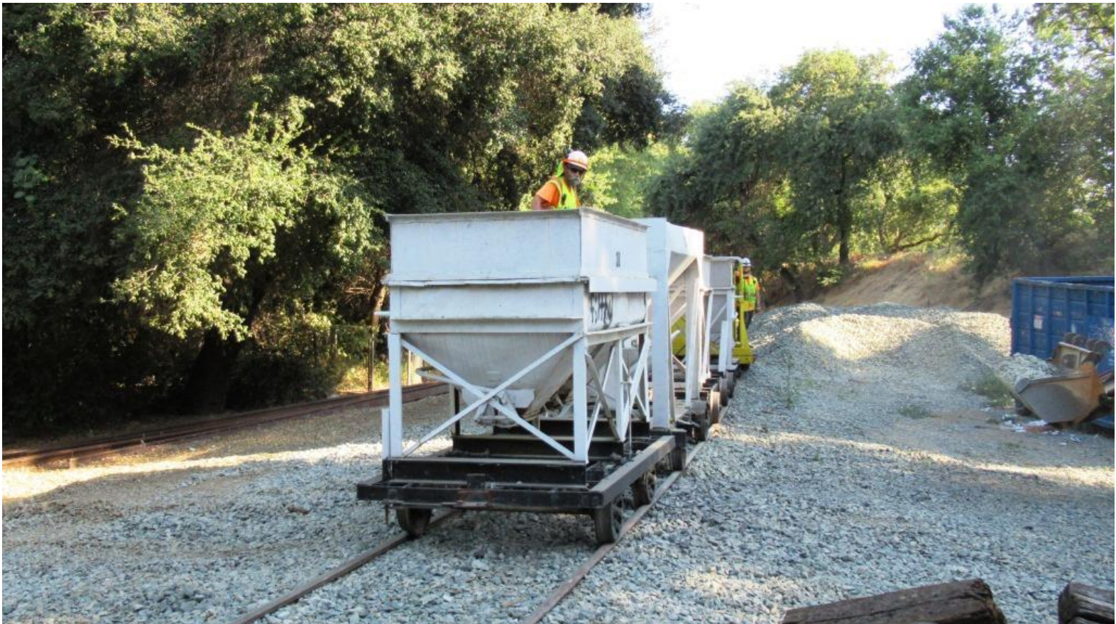
Joe checks the fill-level of the hoppers
