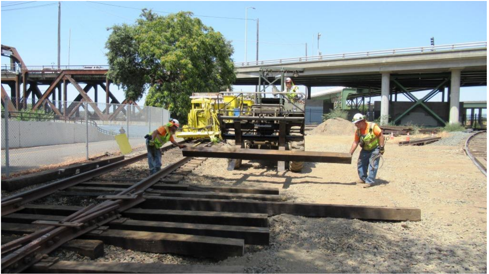
Joe and Mike F. place the long ties that Steve brought over with Big Green
