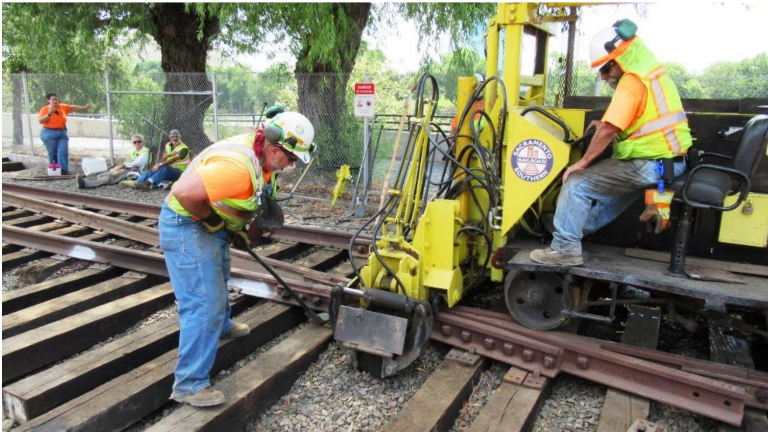
Because the 125's rail-clamps and jack can't grab the frog to lift it, Mike F. tries to nip it up in order to relieve the downward pressure
